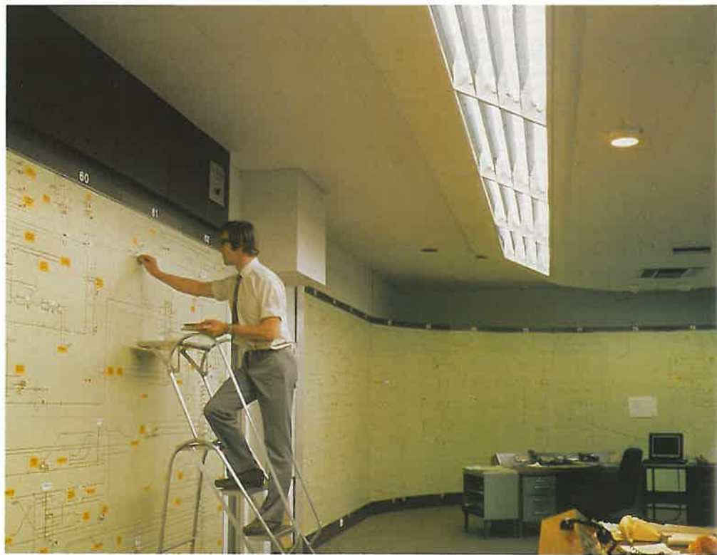
Air-conditioning is a 'must' in this continually manned windowless control room of the EEB at Brentwood, Essex. Air is injected through conventional air diffusers and exhausted through the fluorescent luminaires.
