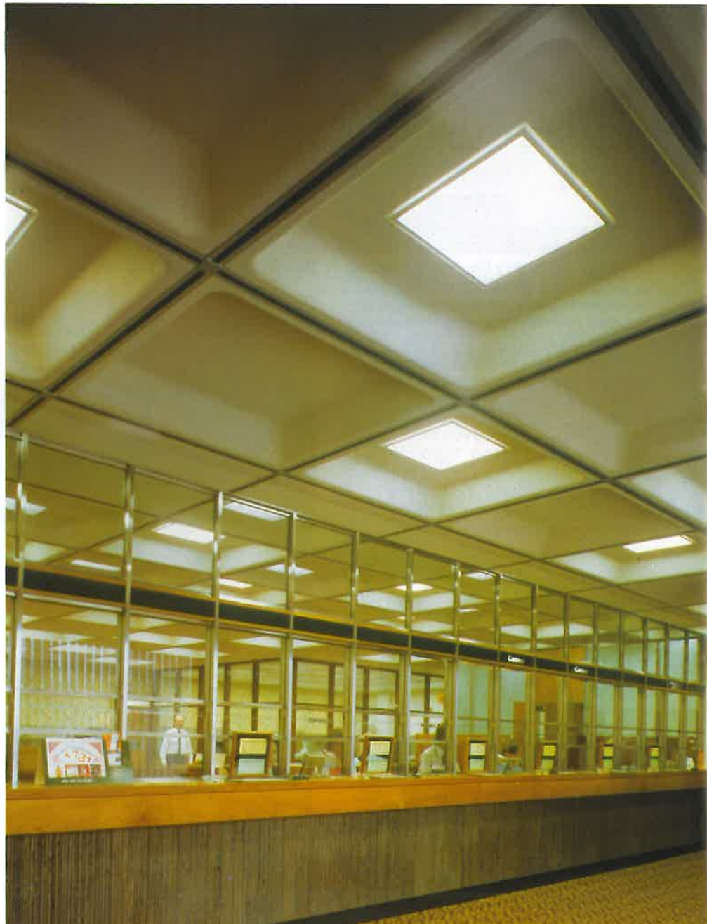
Air-conditioning is a 'must' in this continually manned windowless control room of the EEB at Brentwood, Essex. Air is injected through conventional air diffusers and exhausted through the fluorescent luminaires.
