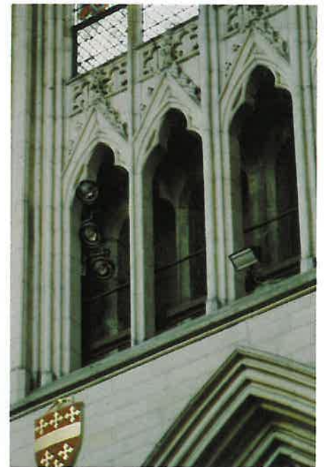
Left: The nave looking east showing the indirect lighting of the vault. The smaller picture shows the arrangement of the 'Sunsports' between the mullions of the triforium. One of the 'Haline' floodlights used for the indirect lighting can be seen in the central opening.
